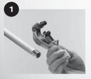
Cut tubing and remove PE coating to expose a minimum of 4 corrugations.
