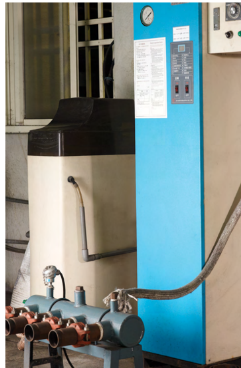
Laboratory hot water testing
